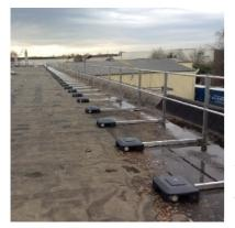
From 3 meters, the law recommends protecting work at height by giving priority to the collective before the individual. The collective protection equipment (CPE) par excellence on flat roofs is the guardrail. This standard or custom-made protective barrier, made of aluminum or galvanized steel, protects against falls from height. It can be installed temporarily or permanently depending on the need.
